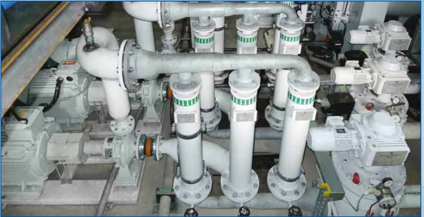
Fig. 6 test water in a steel works
