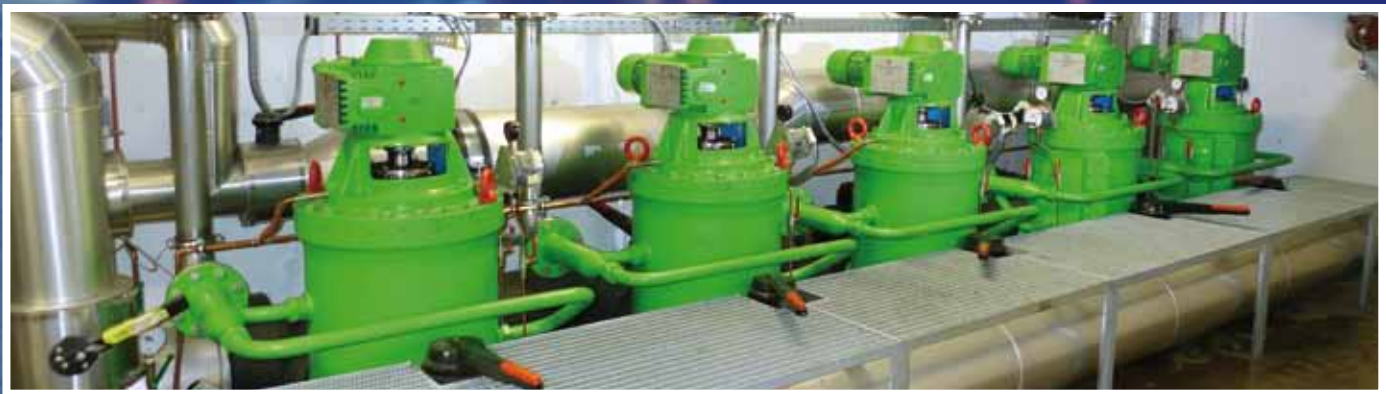
Fig. 18 MUSSEL STOP system at river filtration
