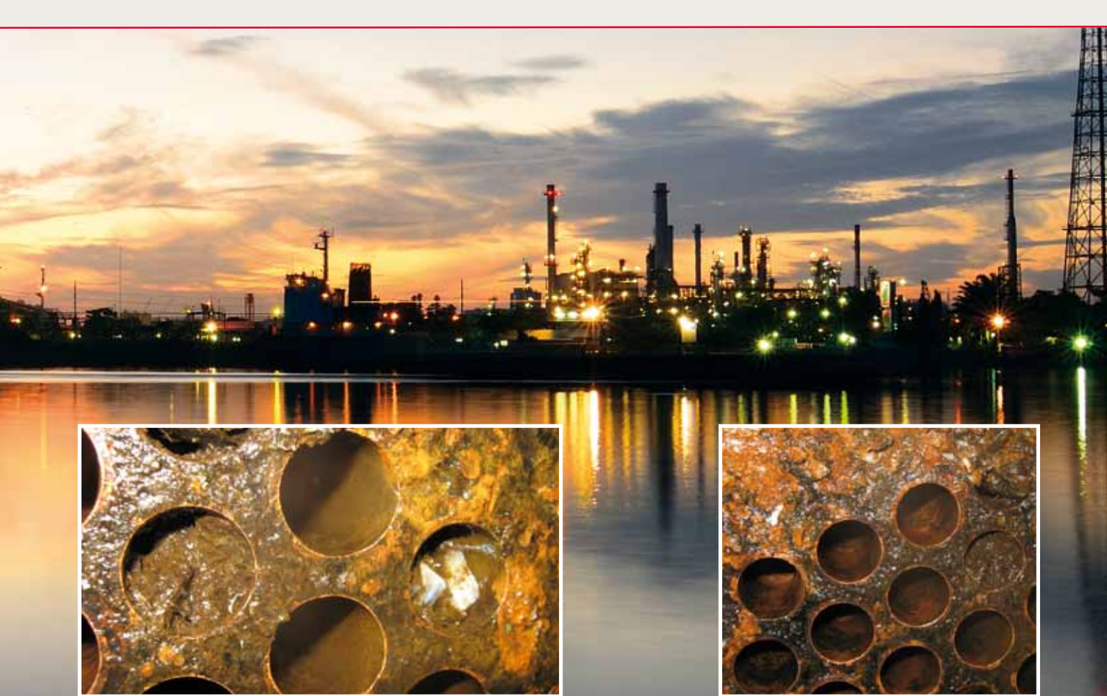
Fig. 7 Mussel infestation of tube heat exchanger
